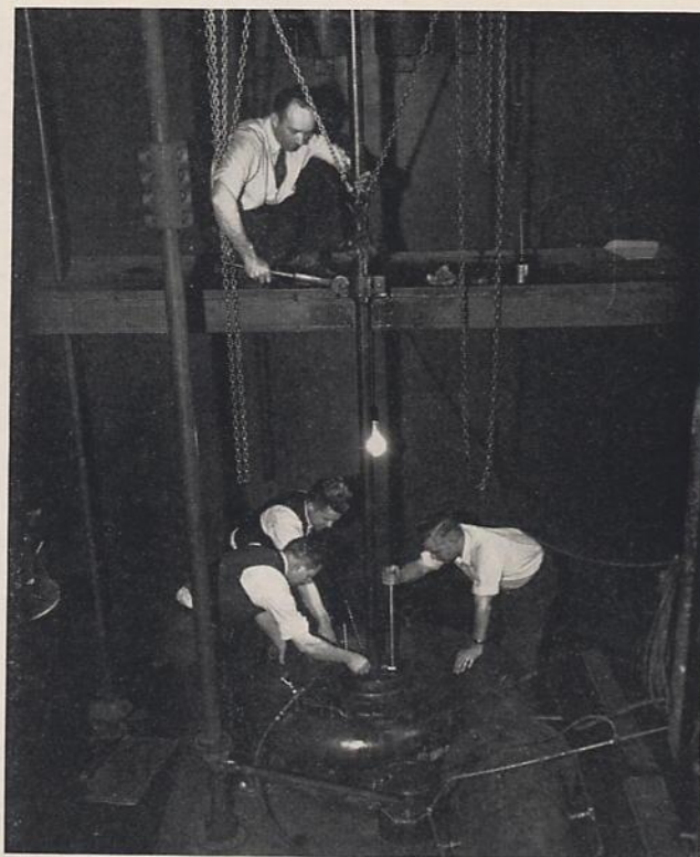
E. G. Latham, K. S. Black, W. C. Madison and C. T. Eagle making final adjustment on Alignment of Turbine Model.
